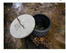
inserted in the hole and the cover, which acts like a stopper, is placed on top. Very shortly the cistern fills with good, clear, clean water that any hiker would be glad to dip into - but should still filter or treat.
